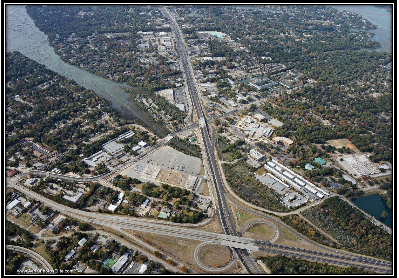
Improvements to Johnnie Dodds Boulevard.
